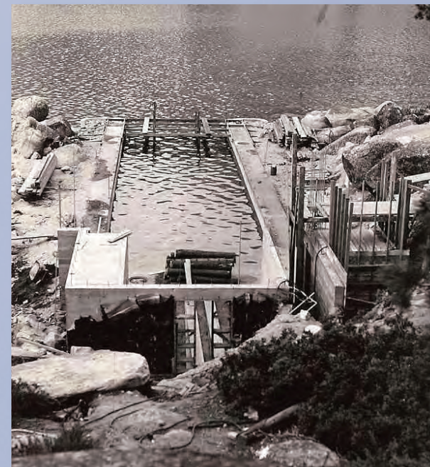
Whittell dynamited a solid granite hillside to construct a concrete and steel boathouse at Lake Tahoe. [Spring 1940]
